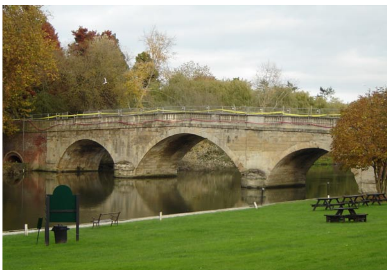
Shillingford Bridge, in the south of Oxfordshire
