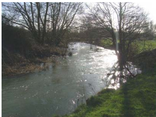
Plate 13: Area of bank erosion (now fenced off)
