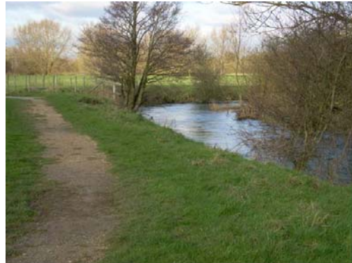
Plate 20: Looking upstream to the bank erosion at the meander bend
