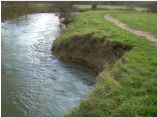
Plate 19: Second eroded bank
