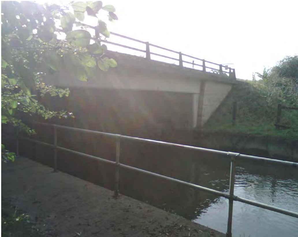
Photograph 5 Structure A upstream face of A40 road bridge
