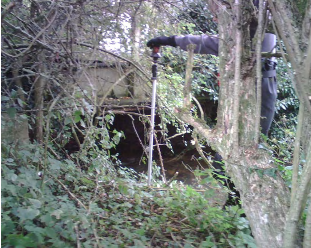
Photograph 11 Structure G upstream face of disused railway bridge
