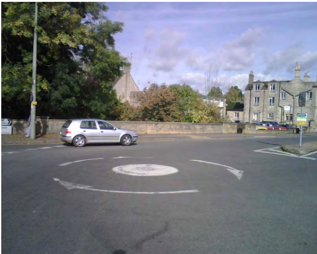
Photograph 8 Structure D Bridge Street road bridge
