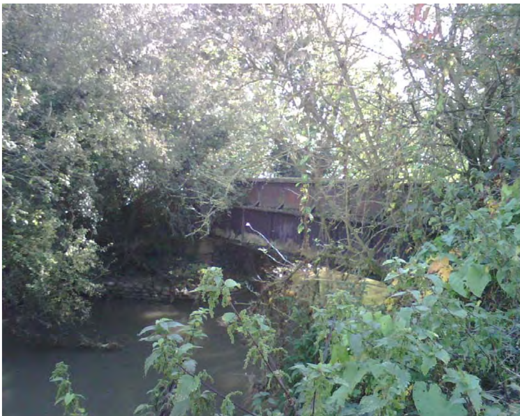
Photograph 6 Structure B upstream face of disused railway bridge
