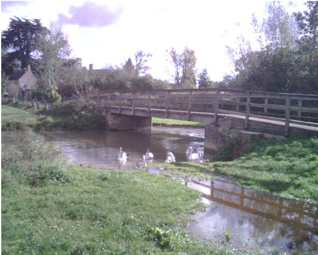
Photograph 13 Structure I upstream face of footbridge
