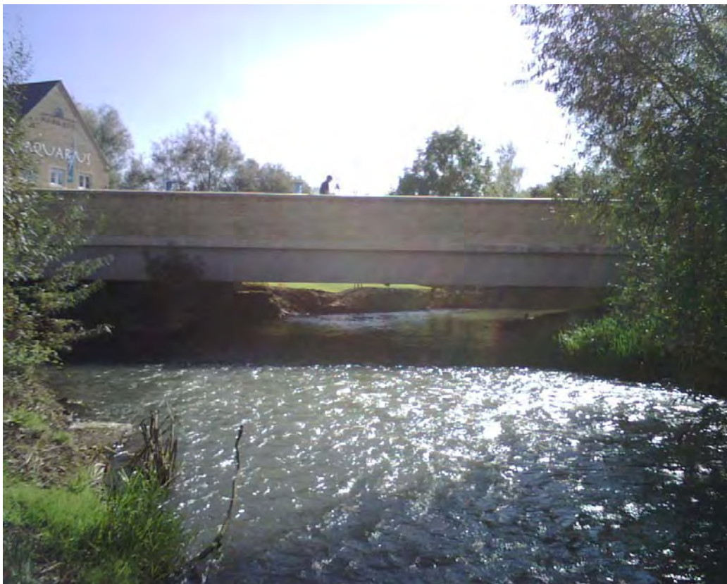
Photograph 4 Structure ST04 upstream face of road bridge
