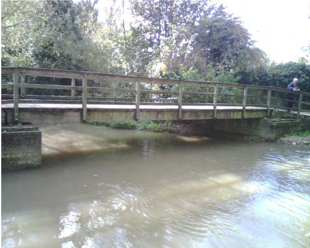
Photograph 7 Structure C upstream face of footbridge
