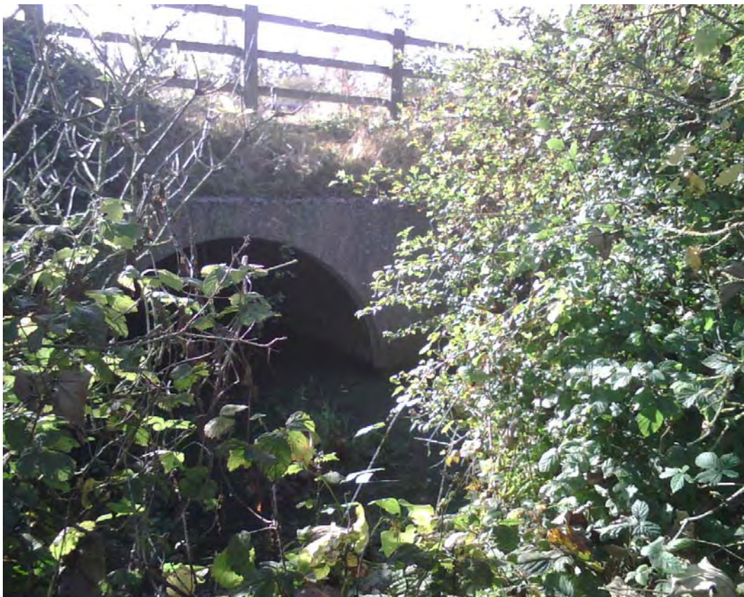
Photograph 14 Structure J upstream face of culvert
