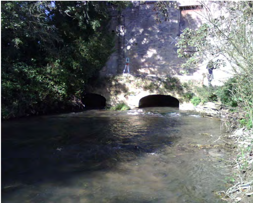
Photograph 19 Cross Section CS5 and downstream face of Farm Mill
