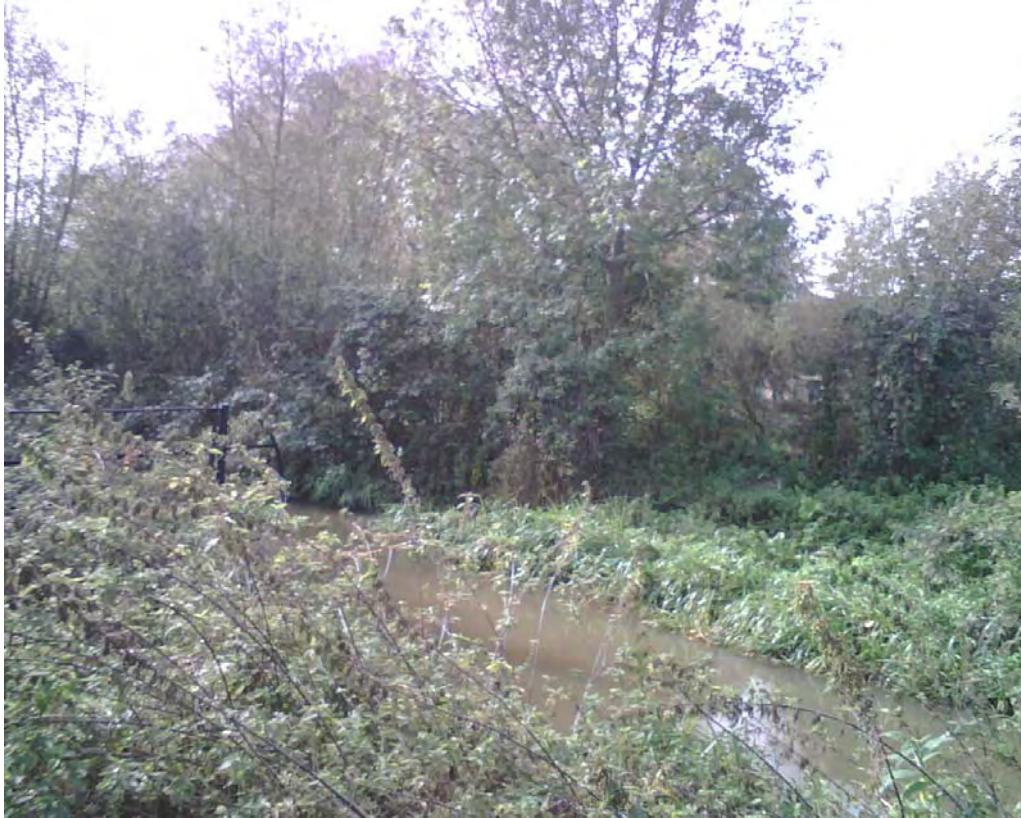
Photograph 1 Structure ST01 Sluice Gate
