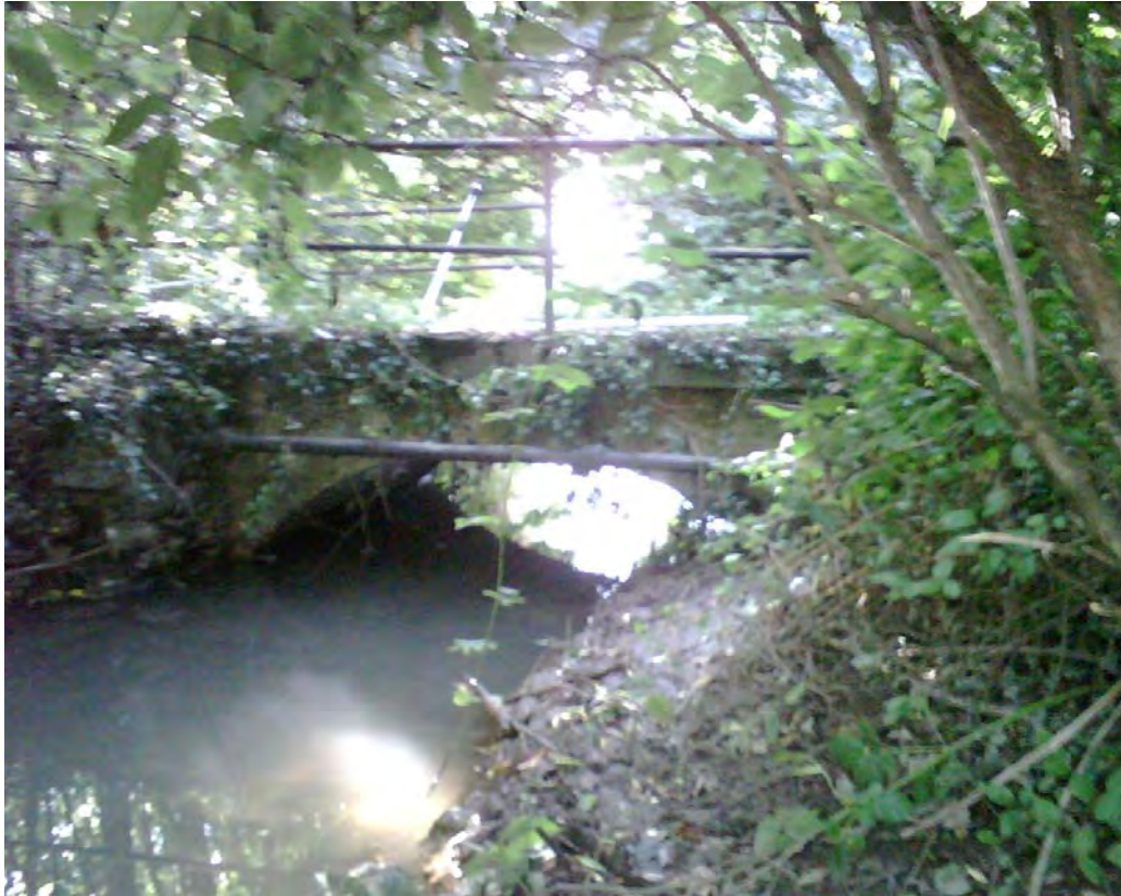
Photograph 3 Structure ST03 upstream face of footbridge
