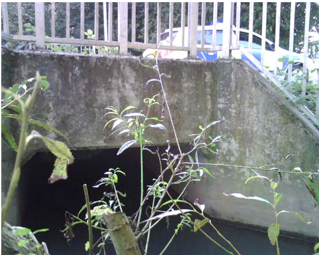
Photograph 2 Structure ST02 upstream face of culvert
