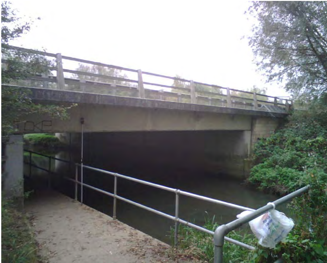
Photograph 9 Structure E upstream face of A40 road bridge
