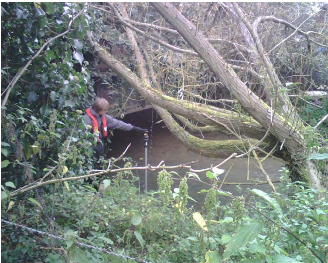
Photograph 10 Structure F upstream face of disused railway bridge
