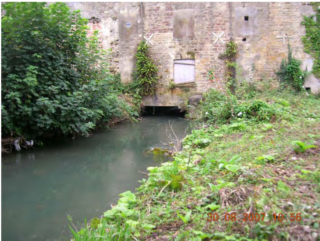
Photograph 12 Structure H upstream face of Farm Mill
