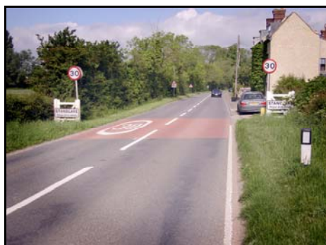
Photo 4 Northbound entry to Standlake showing gateway treatment
