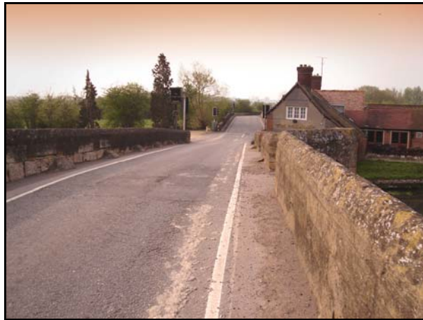
Photo 1 Existing River Thames Crossing at Newbridge
