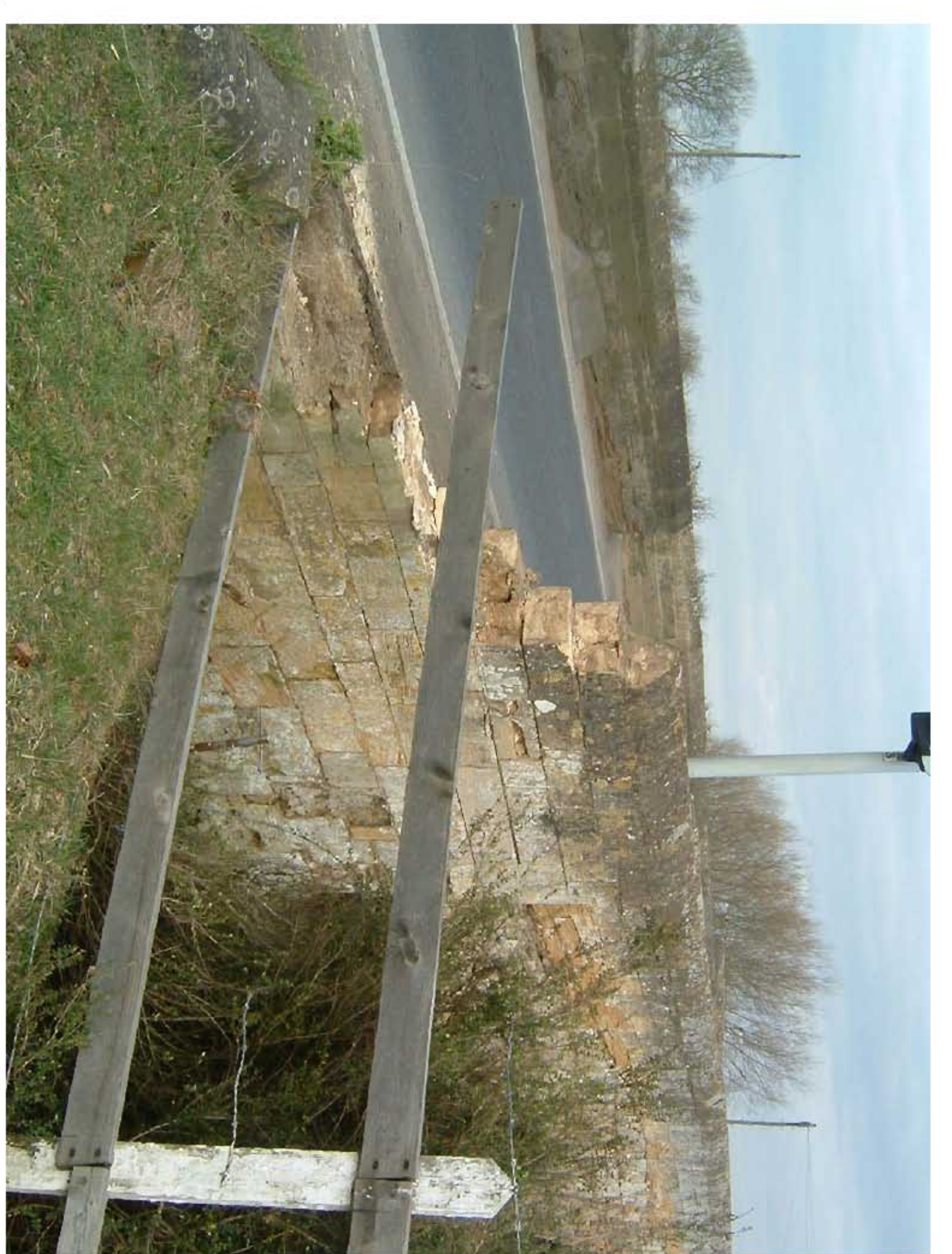
Vehicle Impact Damage to Parapets - 3
