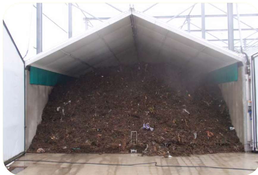
A composting tunnel at Ardley IVC
