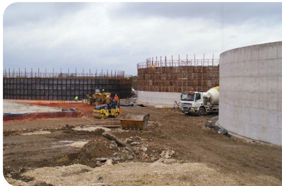
Cassington AD plant under construction
