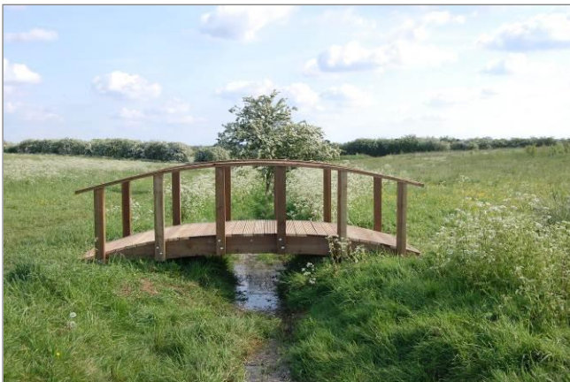
The new footbridge across the stream
