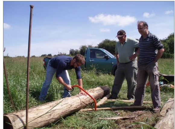
A second footbridge has been made, to a more rustic and simpler design. This is located near the southern entrance gate.
