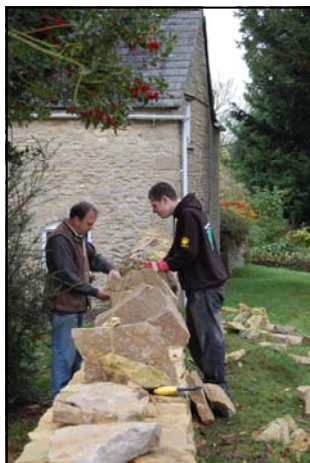
Walling at Fifield Church
