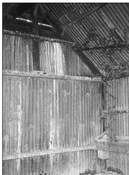
'Whitewash' splashings on a barn end wall
