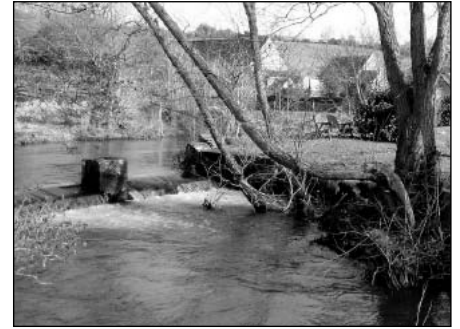
Derelict sluice at Swinbrook
