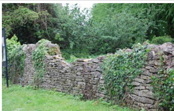
Ascott pound wall... before
