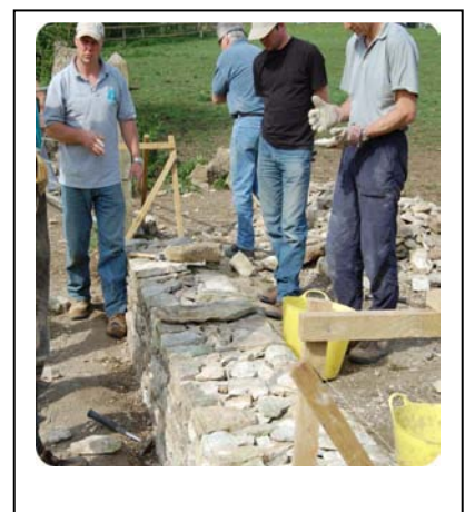
Through stones and galf stones in place
