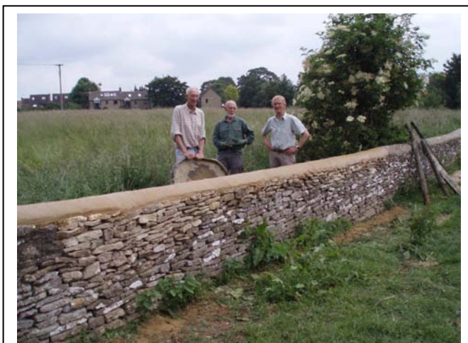
Repairs complete on Langel Common
